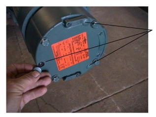
Remove the three plugs on the end of the brake. Tighten each of the three Allen head bolts ¼ turn and try the hoist again. Continue this procedure until the brake works properly.
