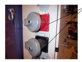
**Blast Motor Plug Receptacle**
