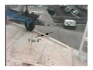
Place the fixture on the roof with the front tires about 3 to 4" from the edge of the tank. Make sure that the fixture is sitting square and that the rear of the fixture is pointed toward the center of the tank.
