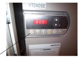
If the speed is above 60 cycle, push the Mode Button and the display will flash showing the A00-0 cycle parameter set point.
