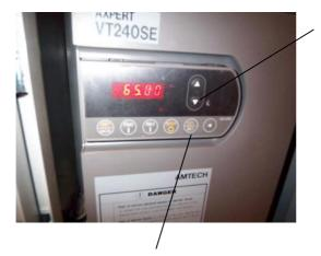
Push the Down Arrow Button to lower the Number, one digit at a time, down to zero. Note: You must change the speed slowly, one digit at a time or the drive will overload.
