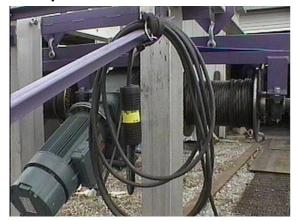
Connect the power cable for the fixture drive to the power cable from the hoist wiring harness. The cable is required to be long for floating roof applications. Roll up the extra cable and secure it to the fixture. Caution- Make sure that all cables are clear of any pinch points and cannot be damaged during operation.
